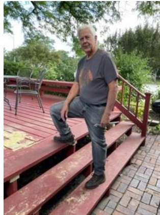
Mike Relaz fixed the risers on the existing deck for the teaching area in the garden.
